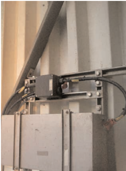
Figure 34: Junction/control boxes and cabinets
