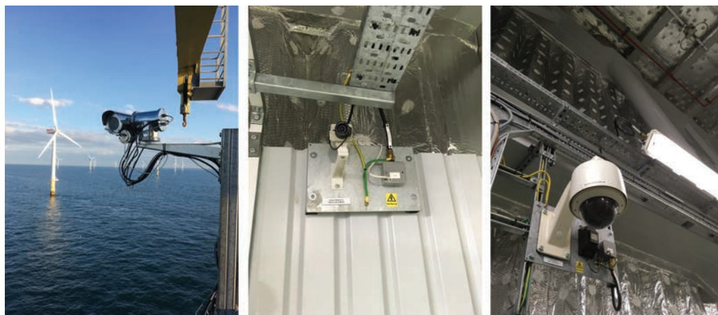
Figure 32: CCTV cameras are subject to dynamic forces, particularly snagging
