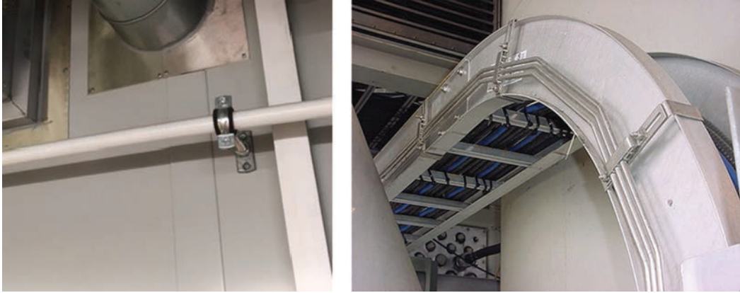
Figure 25: Appropriately engineered pipe clamps should be used
