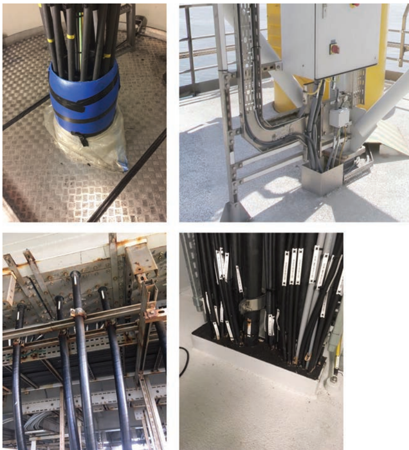
Figure 24: All piping and equipment feedthroughs should have a toe board and should be covered to the greatest extent possible
