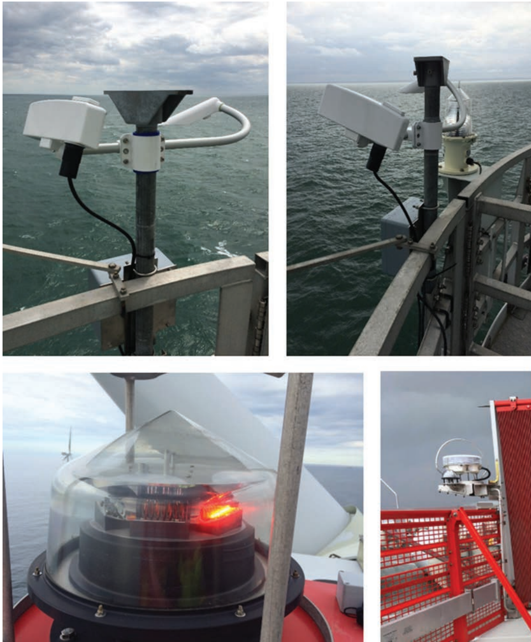
Figure 36: Antennas, lights and sensors are usually mounted at height and are exposed to continuous environmental forces
