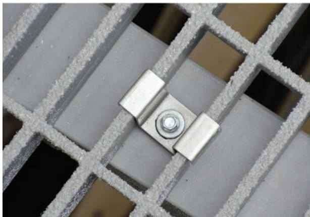
Figure 22: There are a number of different ways of fastening grating to underlying structures or frames
