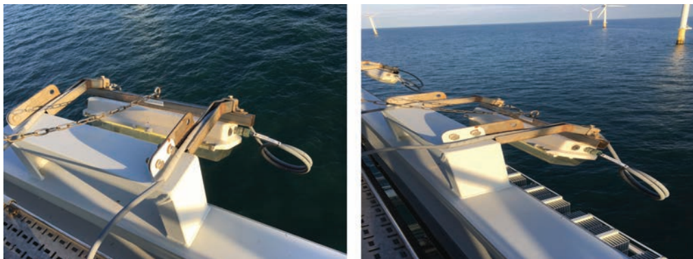
Figure 31: Lighting unit installed at height should be adequately secured against falling or colliding with mobile equipment
