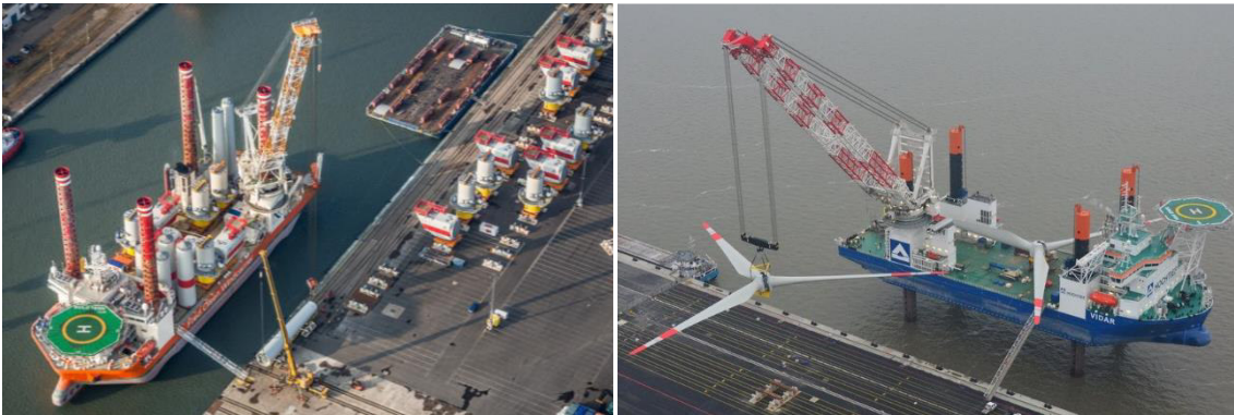
Figure 3-56: JUVs working together on the tower-nacelle and the rotor pre-assembly installations at the Global Tech I wind farm (offshoreWIND.biz, 2014)
