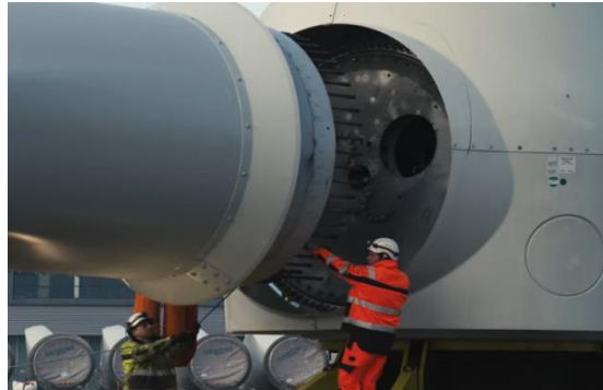
Figure 1-2 Lifting of blade into hub (London Array, 2013)
