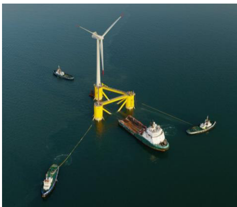
Figure 2-11 Tow out of Principle Power's WindFloat (Bush, 2015)
