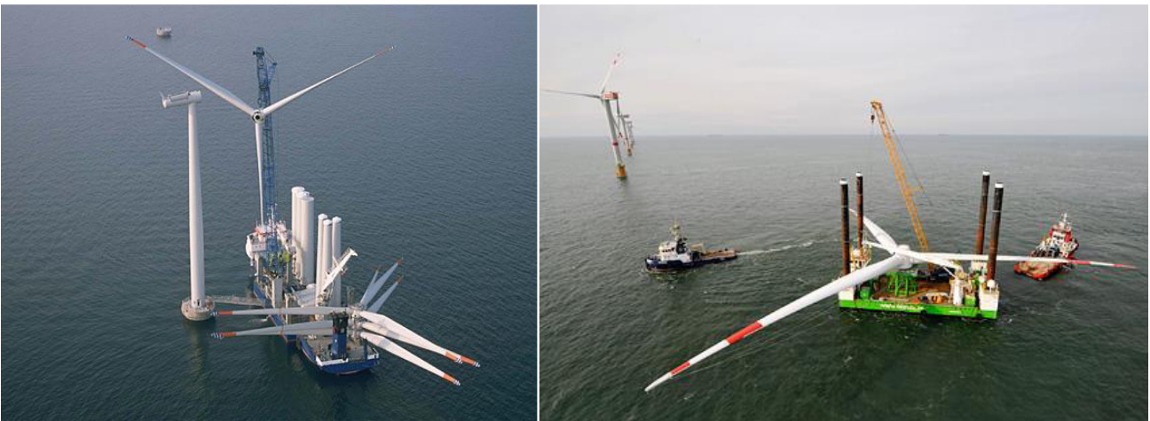
Figure 3-50 ROT configuration offshore installation examples (C-power, 2017; offshoreWIND.biz, 2015)
