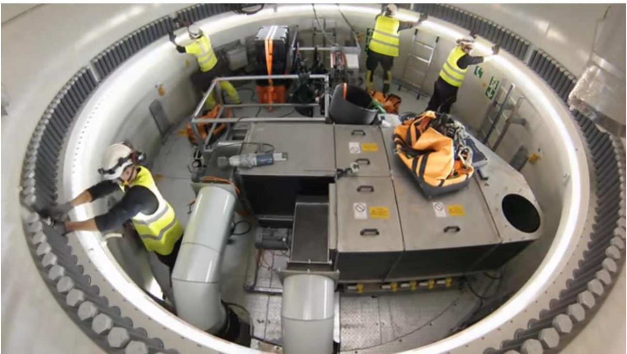
Figure 3-35 View of bolts inside tower section during installation (Fred. Olsen Windcarrier, 2015)
