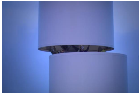
Figure 1-3 Lifting of tower onto transition piece (London Array, 2013)
