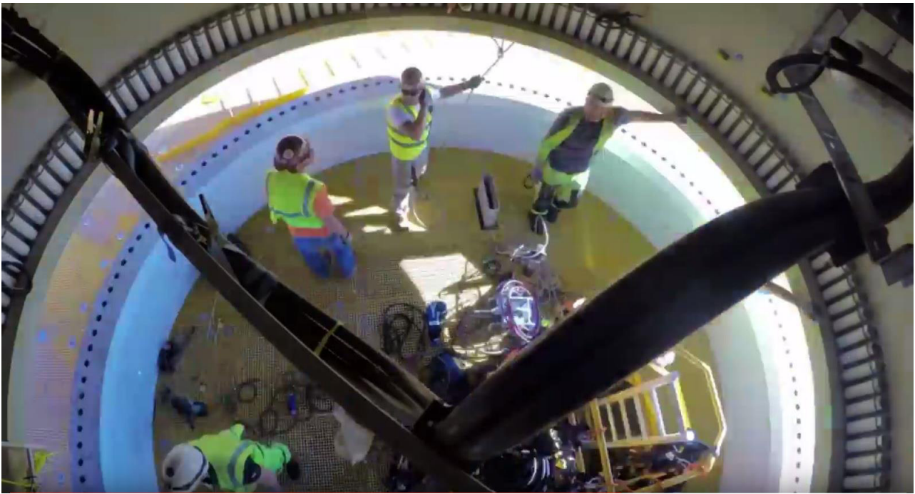
Figure 3-1 People guiding manually the load (Fred. Olsen Windcarrier, 2016b)
