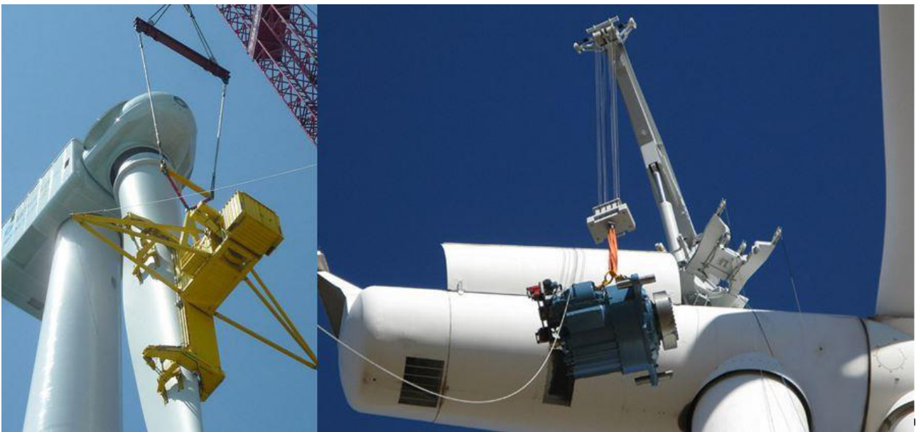
Figure 3-13 Liftra products. Left - Blade Dragon, Right - Self-hoisting crane (Liftra, 2016)
