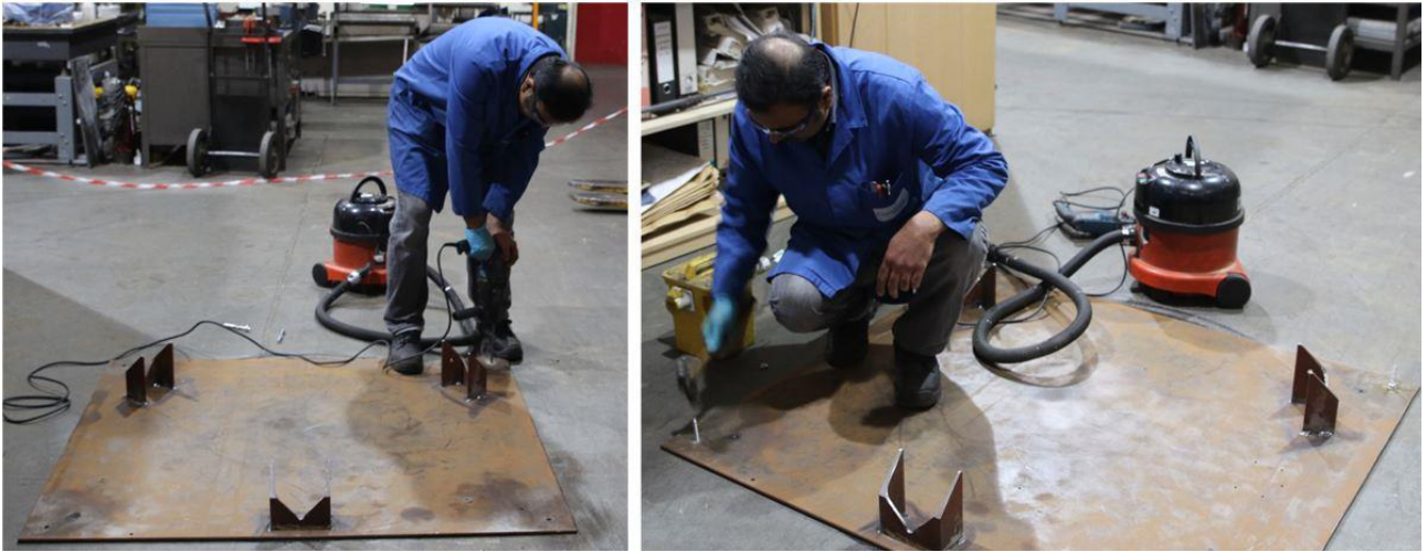
Figure C-7 Fixation of bottom element to floor
