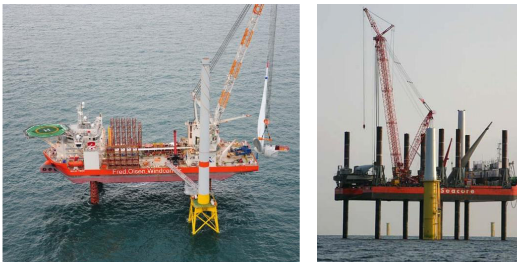
Figure 3-48 Jack-up vessels and barge comparison (during lifting and installation phases of BE pre-assembly) (Fred. Olsen Windcarrier, 2013; Uraz, 2011)
