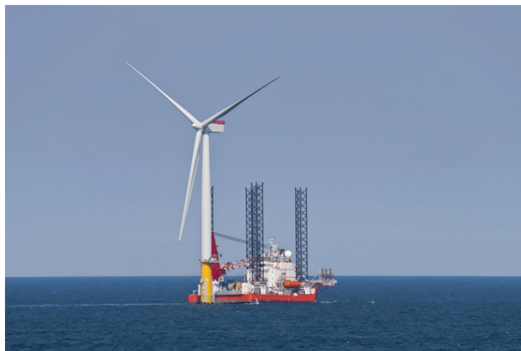
Figure 2: Jack-up vessel next to offshore wind turbine
