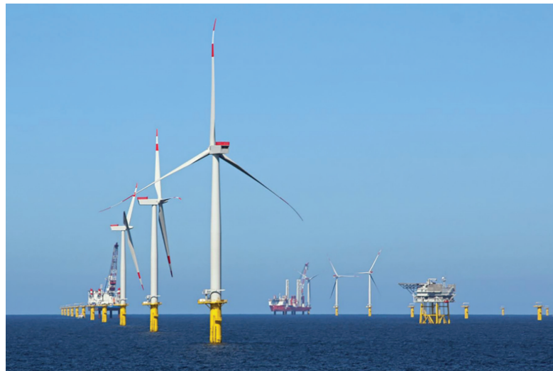
Figure 1: Offshore wind farm in construction
